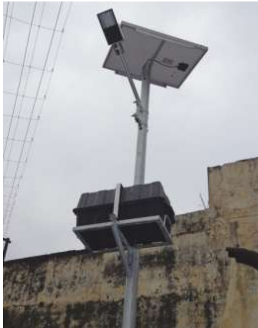
Fig.2.1: Stand Alone LED Solar Light
